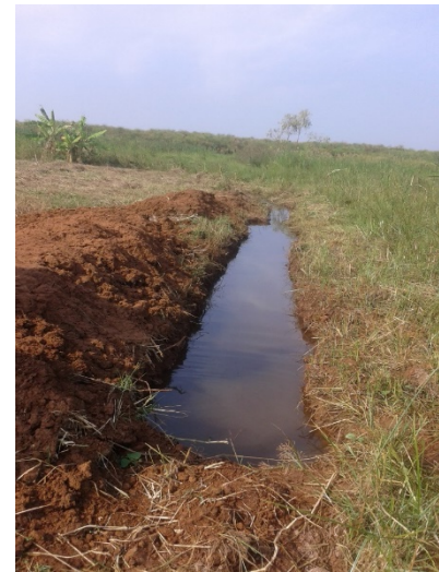
An example of trench within the natural watershed system created for training purpose as part of the KAUW BRPID Project in 2017-2018.
